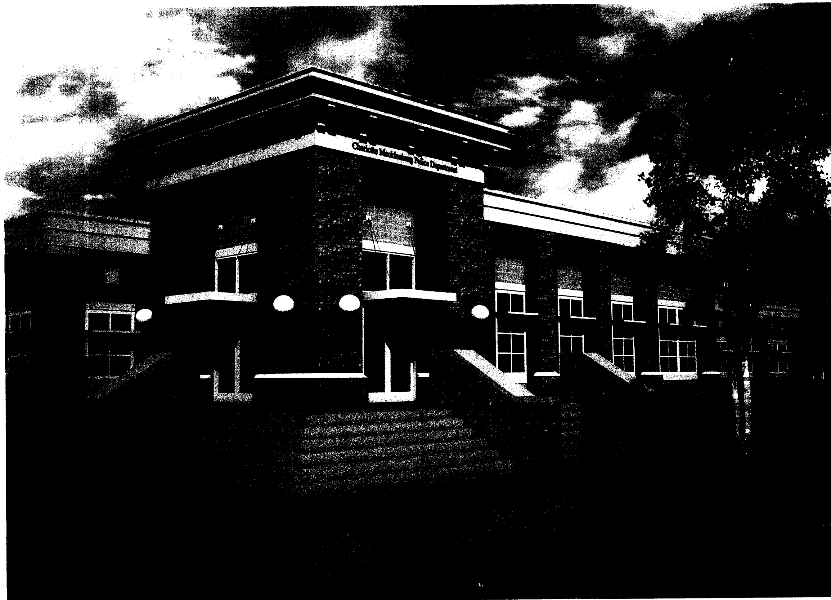
View from corner of Central Ave. and Merry Oaks Rd.
