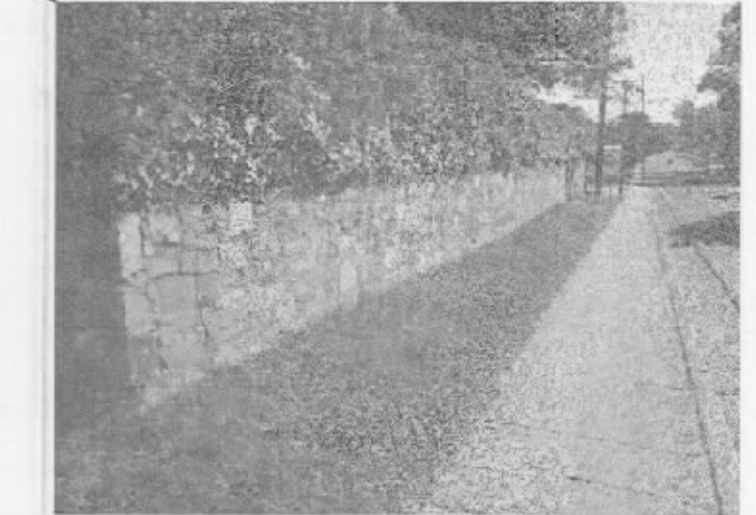
EXISTING RETAINING WALL AND SIDEWALK
