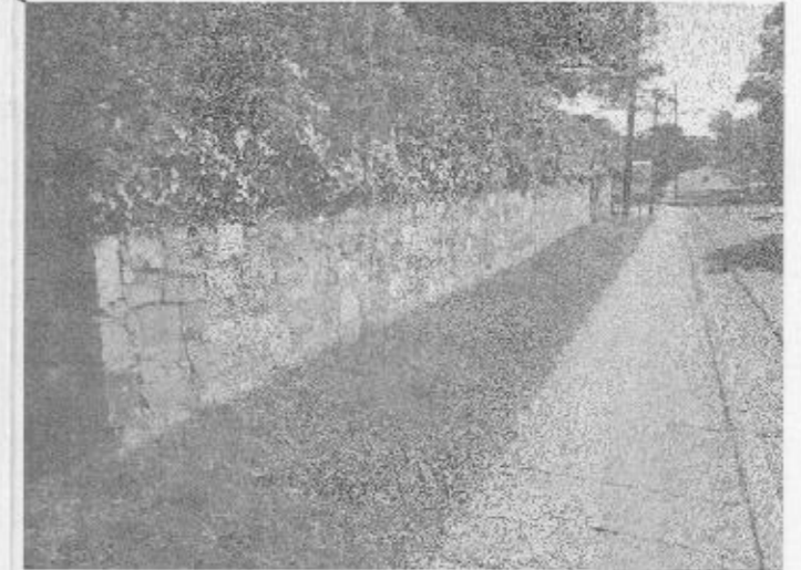
EXISTING RETAINING WALL AND SIDEWALK
