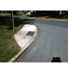
X Walk 1 Slope (%) 2.0 X Walk 2 Slope (%) N/A X Walk 1 X Slope (%) 2.7 X Walk 2 X Slope (%) N/A N/A N/A Ramp inside XWalk2? Ramp inside XWalk1? N/A Road Slope (%) 2.7 Clear Space? N/A Road X Slope (%) 2.0 N/A Clear Space to XWalk (in) N/A N/A N/A N/A Any Obstructions? Storm Grate/Utility Hazard? N/A **Obstruction Type** 3200.00 Storm Grate/Utility Type N/A N/A Yes Surface Condition? (G/P) Good No 7.1 Curb Slope (%)
