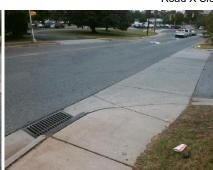
Road X Slope (%) 1.1 N/A Clear Space to XWalk (in) N/A N/A Any Obstruction? N/A **Obstruction Type** N/A N/A Storm Grate/Utility Hazard? N/A Storm Grate/Utility Type N/A Yes Surface Condition? (G/P) Good Curb Slope (%) 5.5
