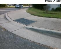
X Walk 1 X Slope (%) 2.5 X Walk 2 X Slope (%) 5.0 N/A 3200.00 N/A Ramp inside XWalk1? N/A Ramp inside XWalk2? N/A Road Slope (%) 1.5 Clear Space? N/A Road X Slope (%) 3.8 N/A Clear Space to XWalk (in) N/A N/A Any Obstruction? N/A **Obstruction Type** N/A N/A Storm Grate/Utility Hazard? N/A Storm Grate/Utility Type N/A Yes Surface Condition? (G/P) Good 20.1 Curb Slope (%)
