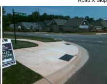
X Walk 1 Width (in) N/A X Walk 2 Width (in) N/A X Walk 2 Slope (%) 3.5 N/A X Walk 1 Slope (%) X Walk 1 X Slope (%) 10.7 X Walk 2 X Slope (%) N/A 1800.00 N/A Ramp inside XWalk1? N/A N/A Ramp inside XWalk2? N/A Road Slope (%) N/A Clear Space? N/A Road X Slope (%) N/A N/A Clear Space to XWalk (in) N/A N/A Any Obstruction? N/A **Obstruction Type** N/A N/A Storm Grate/Utility Hazard? N/A Storm Grate/Utility Type N/A Yes Surface Condition? (G/P) Good 12.0 Curb Slope (%)
