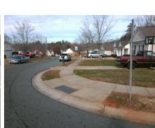
No Painted X Walk2? N/A To S X Walk 2 Direction N/A N/A X Walk 2 Width (in) N/A 4.8 X Walk 2 Slope (%) N/A 3.5 X Walk 2 X Slope (%) N/A N/A N/A Ramp inside XWalk2? N/A 3.5 Clear Space? N/A N/A Clear Space to XWalk (in) N/A 4.8 N/A N/A Storm Grate/Utility Hazard? N/A Storm Grate/Utility Type N/A N/A Yes Surface Condition? (G/P) Good No Curb Slope (%) 20.4
