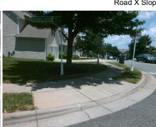
N/A 3200.00 N/A Ramp inside XWalk1? N/A Ramp inside XWalk2? N/A Road Slope (%) 1.6 Clear Space? N/A Road X Slope (%) 4.6 N/A Clear Space to XWalk (in) N/A N/A Any Obstruction? N/A **Obstruction Type** N/A N/A Storm Grate/Utility Hazard? N/A Storm Grate/Utility Type N/A Yes Surface Condition? (G/P) Good N/A Curb Slope (%)
