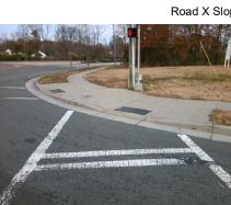
X Walk 1 X Slope (%) 1.5 X Walk 2 X Slope (%) N/A 2550.00 Yes Ramp inside XWalk1? Yes N/A Ramp inside XWalk2? N/A Road Slope (%) N/A Clear Space? Yes Road X Slope (%) N/A N/A Clear Space to XWalk (in) N/A Yes Any Obstruction? No **Obstruction Type** N/A Yes Storm Grate/Utility Hazard? No Storm Grate/Utility Type N/A Yes Surface Condition? (G/P) Good 16.9 Curb Slope (%)
