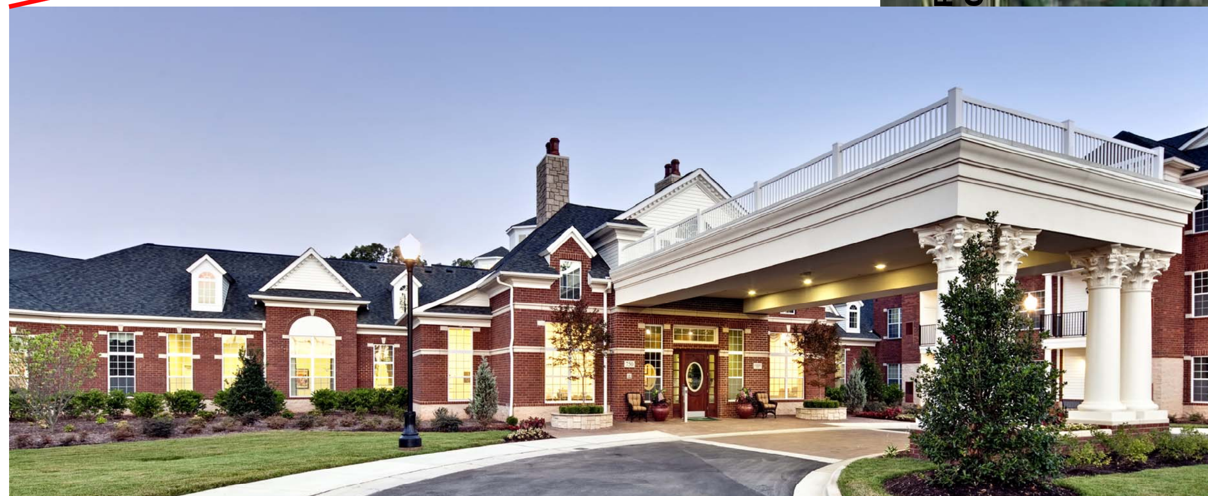
WALTONWOOD CARY, N.C. 1-STORY MAIN ENTRANCE **WALTONWOOD PROVIDENCE COUNTRY CLUB SHALL BE 1-STORY**
