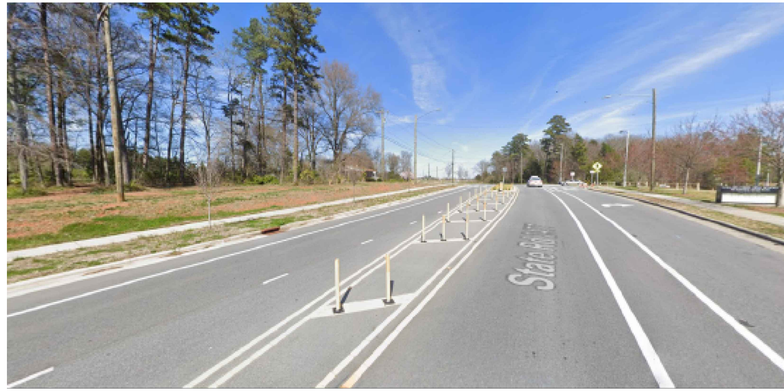
EXISTING STRIPING AND CONTROLLED ACCESS PADDLES ALONG JOHNSTON OEHLER ROAD
