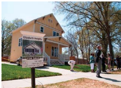
District 1 Orange and Heflin Streets New Construction
