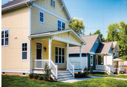
District 2 1000 Rodey Ave. 1001 & 1101 Holland Ave. New Construction
