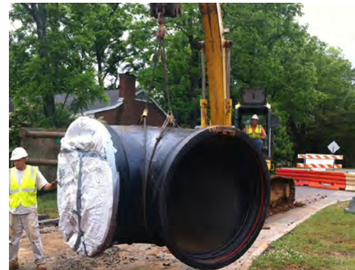
60- and 36-inch Statesville Road Water Line Extension
