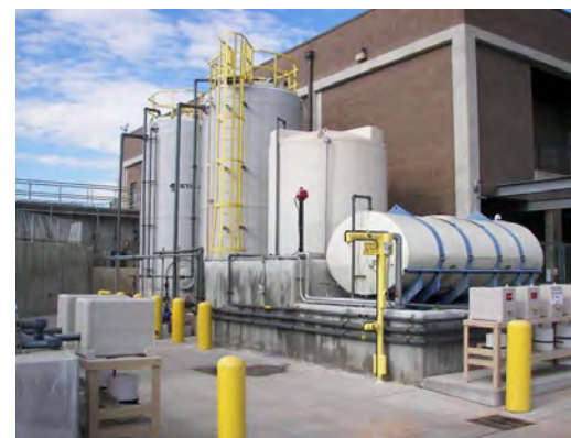
Broad River Water Authority Water Treatment Plant Expansion
