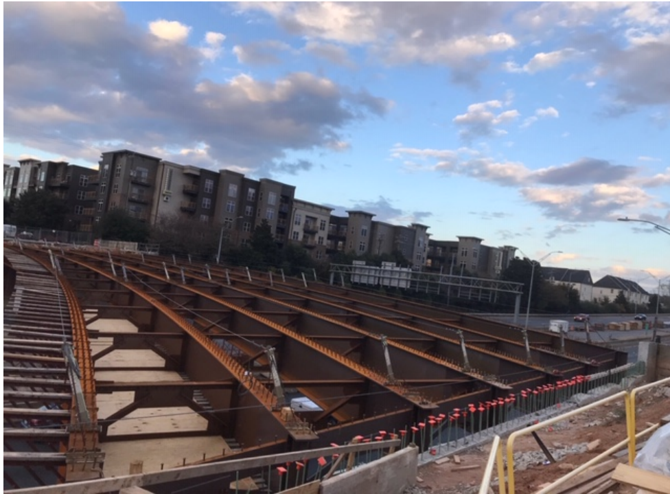
New Bridge Girders installed
